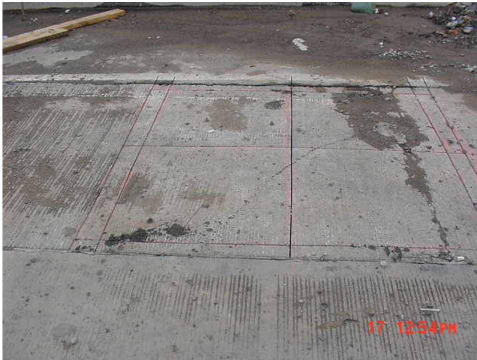
THE SAW CUTS FOR THE LIFTOUT METHOD
