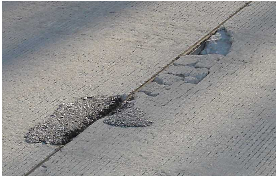
SPALL AT TRANSVERSE JOINT
