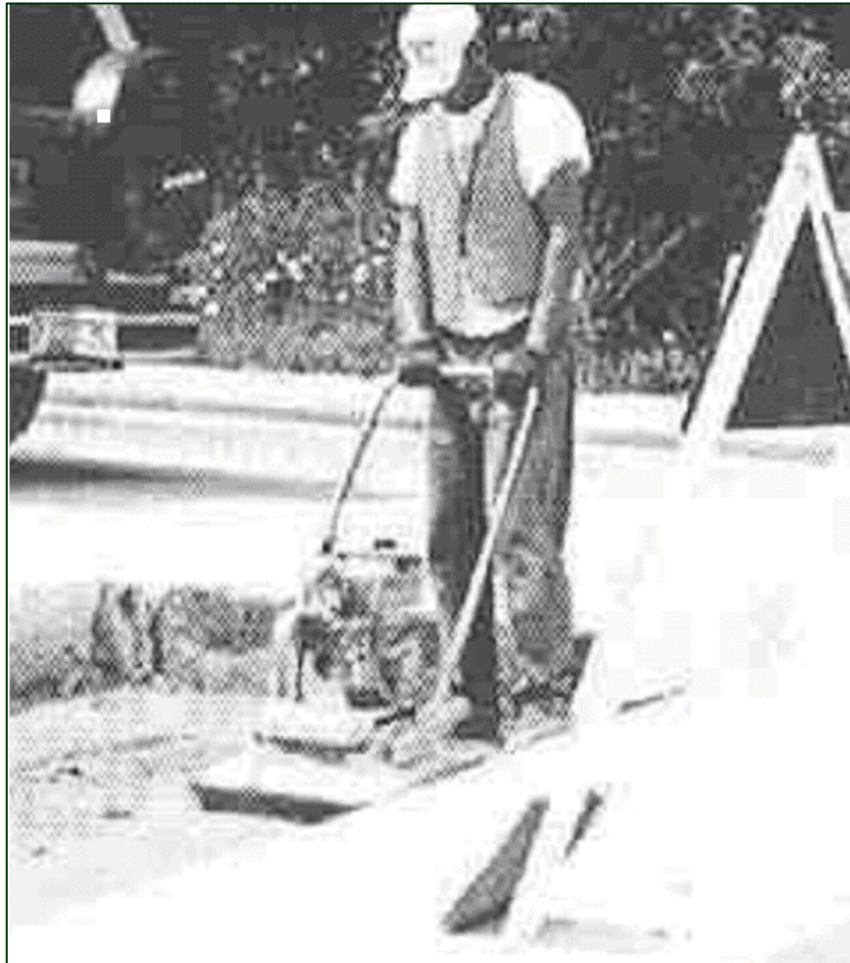
REPAIRING THE BASE LAYER
