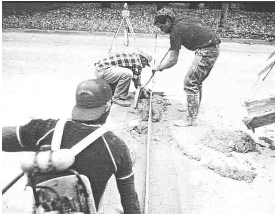
PLACING REPAIR MATERIAL WITH COMPRESSIBLES IN JOINT LOCATION
