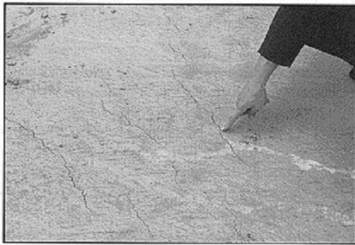
Plastic Shrinkage Cracks
