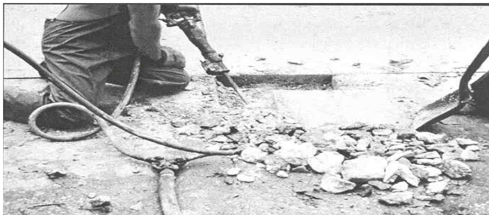
REMOVING THE UNSOUND CONCRETE
