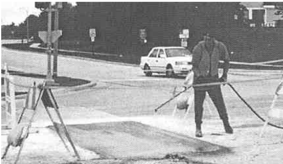
Protect the Repair From Rapid Evaporation
